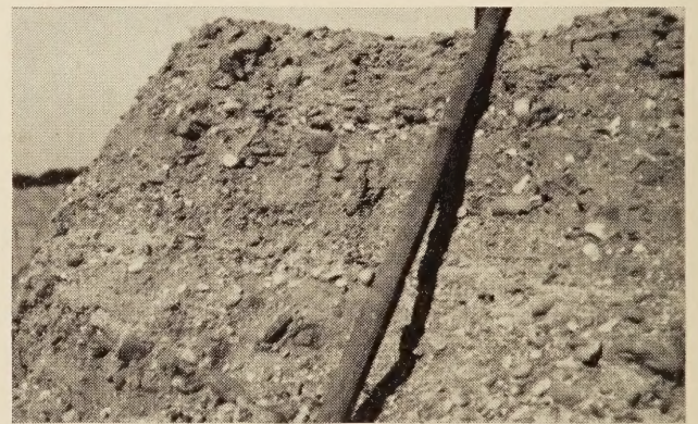
FIGURE 3.—TYPICAL FORMATION OF GRAVEL DEPOSITED BY PUMPING OPERATIONS.
